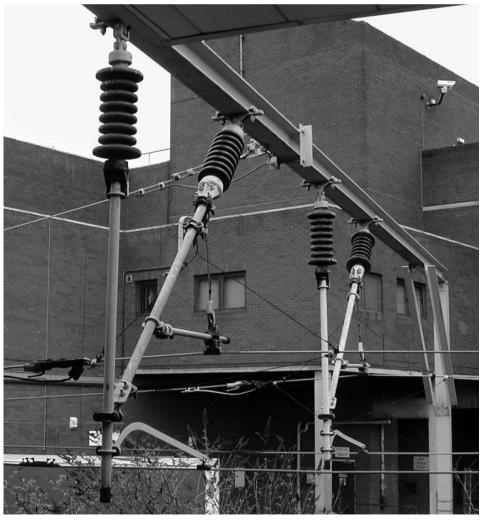
Above: Close up of cantilevers at Walsall Although the arrangement of the Cantilevers is highly variable the parts themselves seem pretty standard. Photo Jim Smith-Wright
