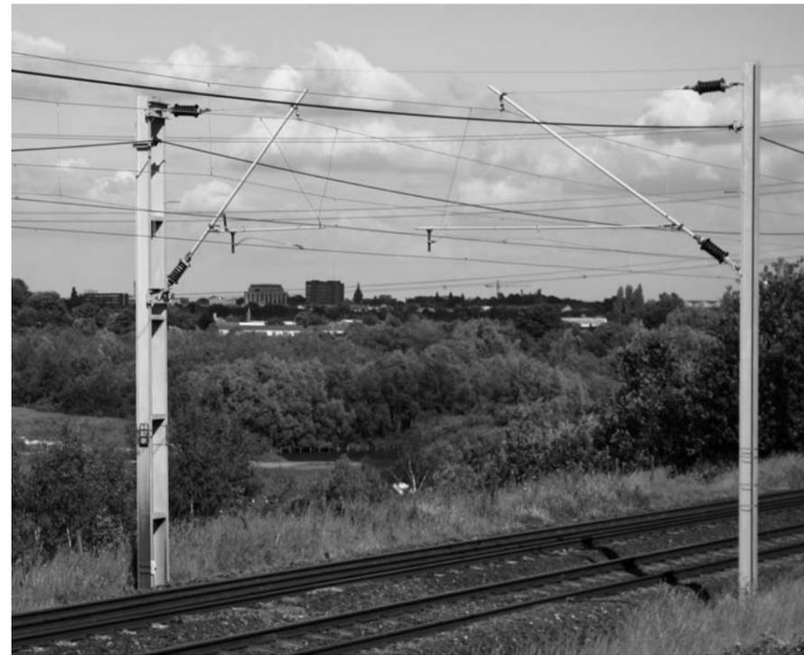
Above: *It may well be that there is no such thing as a standard OLE mast. This pair are at Dudley Port and show the early design MK1 mast on the right. This is a 3 wire system but the auxiliary catenary wire is unrestrained by the cantilevers. Compare the positioning of the earth wire with the drawing on page 34. Photo Jim Smith-Wright*
